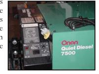
Prior to starting or stopping the generator, make sure that all the 120 VAC appliances are turned Figure 7-17. Electrical Generator
