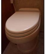
toilet operates with water from either the fresh water tank with the water pump "on" or the city water supply. Before using the toilet, add water to the bottom of the tank. Refer to the "BLACK WATER TANK" instructions elsewhere in this chapter. The toilet flushes waste directly into the black-water holding tank. The toilet uses high-velocity water injection to produce swirl effect in the bowl.
