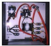
Figure 7-19. Resettable Circuit Breakers
