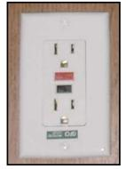
Figure 7-14. Ground-Fault Circuit Interrupter (GFCI)
