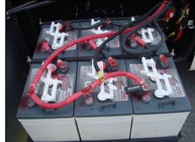
Figure 7-6. Battery Slide Tray
