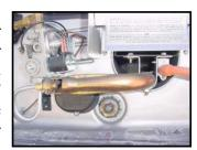
Figure 4-16. Water Heater Drain
